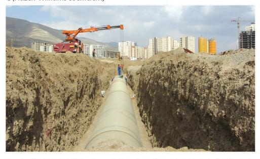
Due to the fact that the closest diameter of Faratec pipes to 1777mm is 1800 mm, a pipe with this diameter will be used. While the internal roughness of the metal pipes increases with time, the roughness of Faratec pipes is constant over time.
