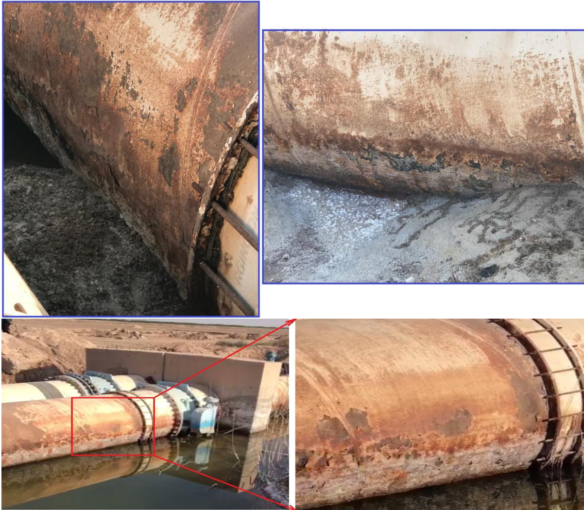
Fig.2.1. Sample of Steel Pipes High Corrosion (Khuzestan Province)
